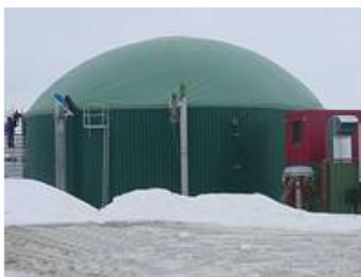
Figure 4: Gas storage with foil memory [Source: Agrotel]
